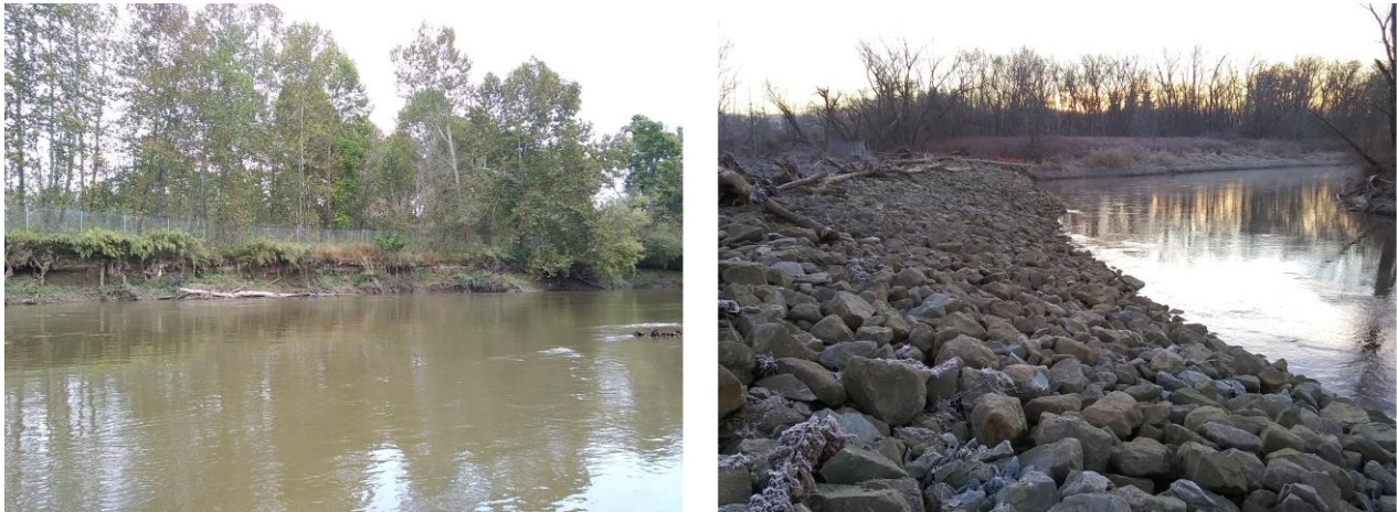
Figure 17. Riprap Revetment Example Before and After Construction
