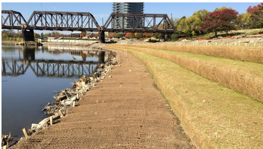
Figure 16. Reinforced Bank Example Under Construction
