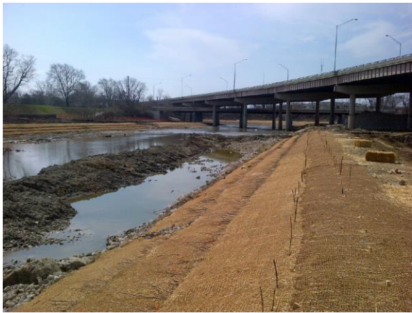
Figure 15. Bioengineered Bank During and After Construction
