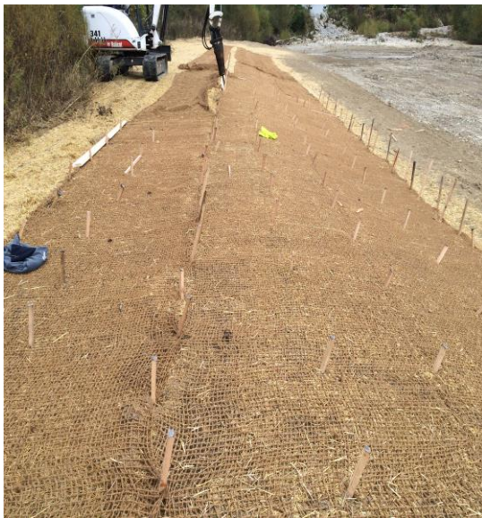
Figure 14. Revegetation Example During and After Construction
